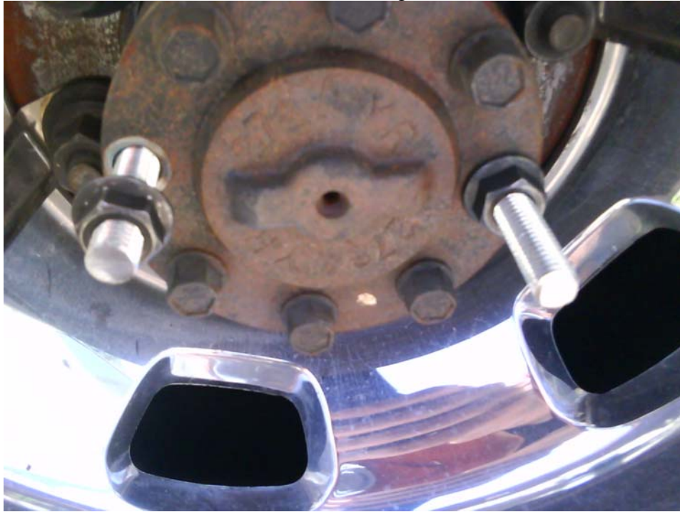
Photo 3: Installing Axle Flange Nuts
